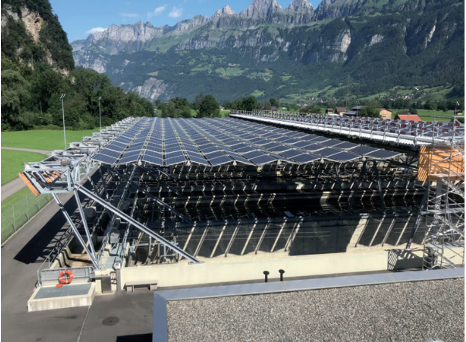
Solarfaltdachanlage
